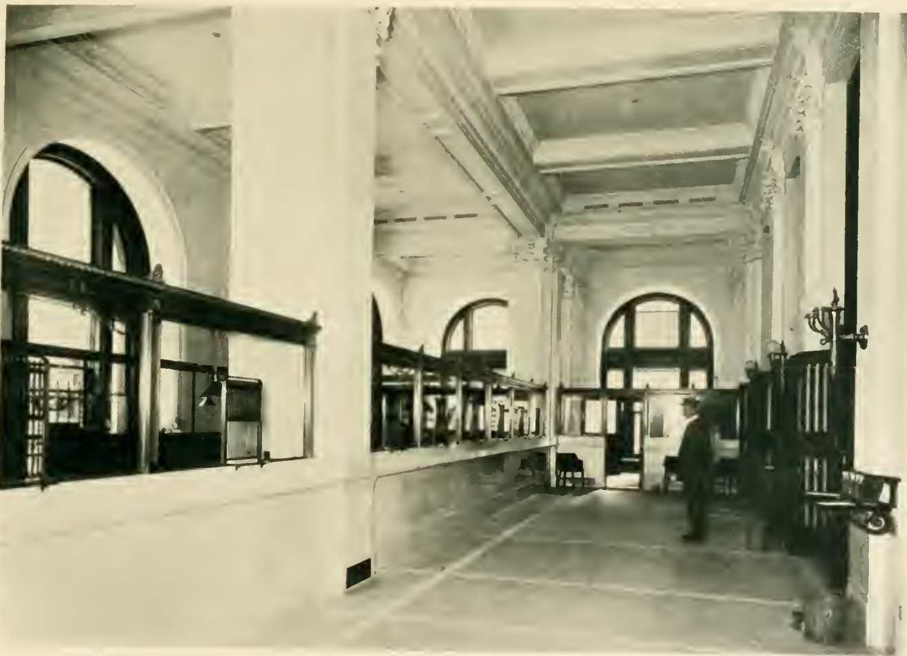
INTERIOR OF BANK, LOOKING WEST.
